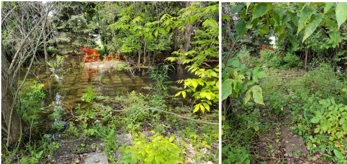
Photos: Left – Outlet weir in Paradise Park 5-30-19, Right – Outlet weir 9-10-19
