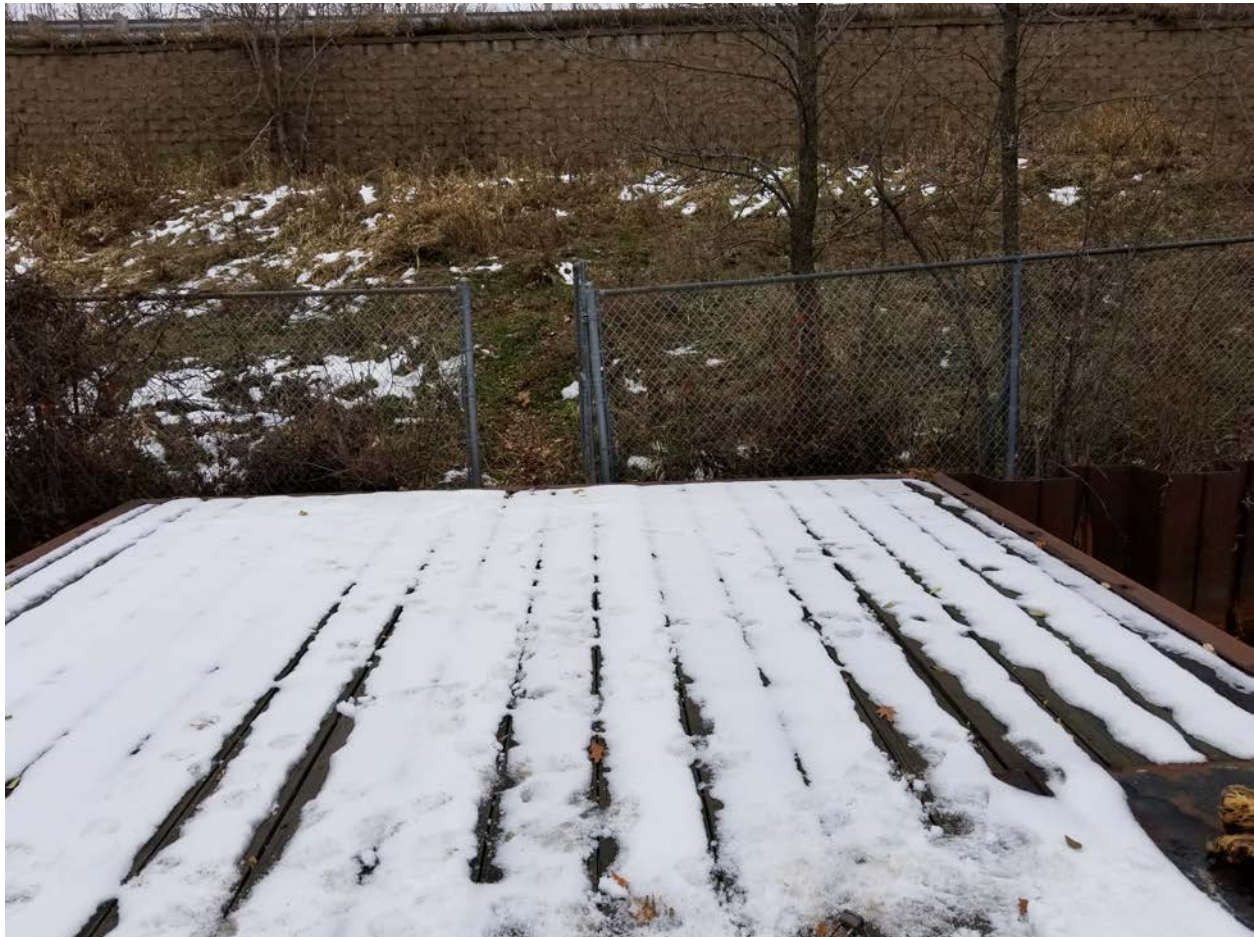
Photos: Outlet Control Structure
