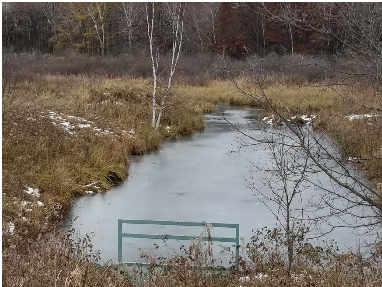
Photo: Ivywood Control Structure
