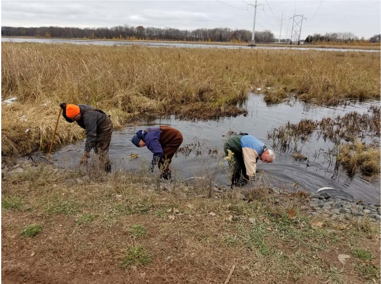
Photo: removing rocks from outlet pipes at Swamp Lake
