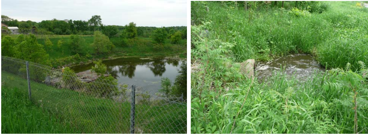
Photos: Left: Outlet Structure, Right: Water flowing to Green Lake
