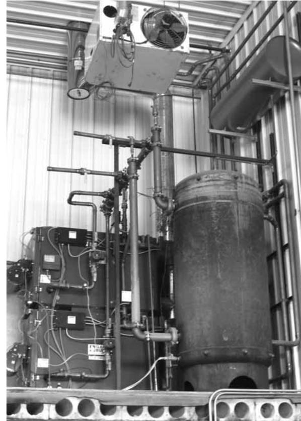
A special new furnace at SRC burns used motor oil to heat its recycling center building in winter, saving thousands of dollars in fuel costs annually.
