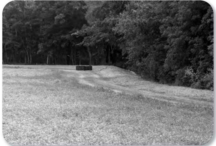
A water and sediment control basin used to stabilize a gully downstream. The large berm holds water back and a pipe slowly releases water into a controlled channel.
